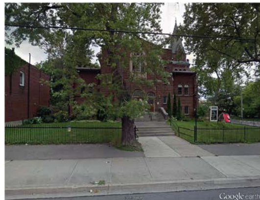
Plate 12: Looking N from Mimico Ave right-of-way (from Google Earth 2013 Streetview)
