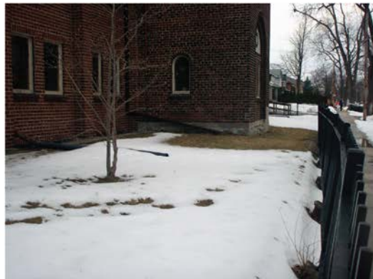
Plate 6: Looking N from SE corner of church - note grade
