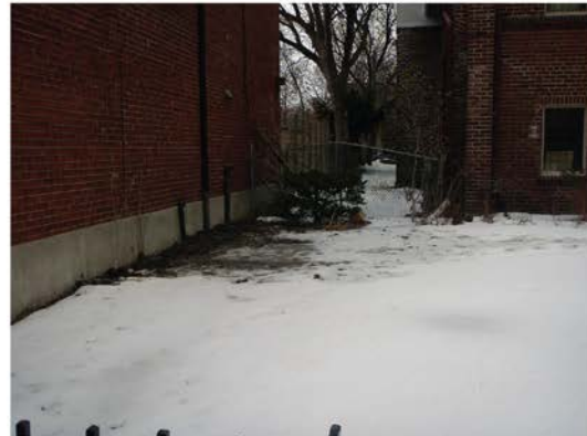
Plate 10: Looking N from SW corner - note grade
