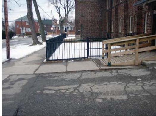
Plate 2: Looking S from NE corner of church - note grade
